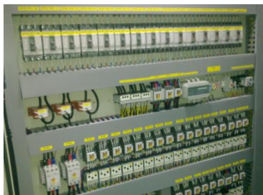
PLC, MCC, Wiring work & Control system
