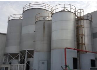
Tanks & Pipeline Installation
